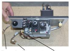
Thermopile Thermocouple Pilot Nut Wire Wire
